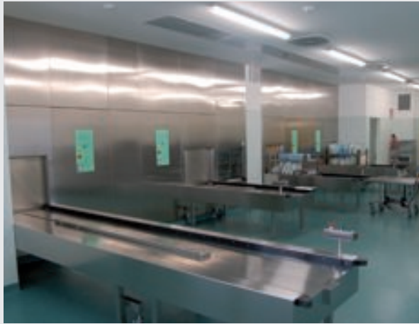
Sterilization unloading side
