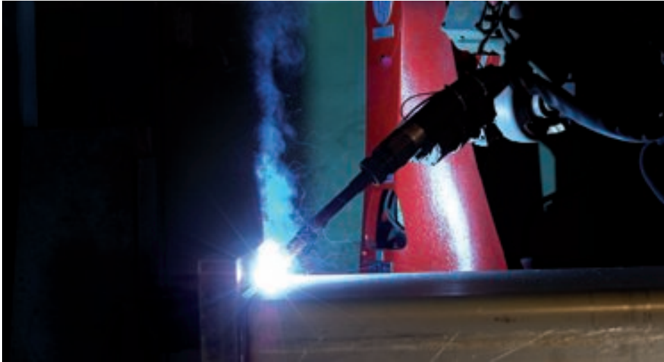
Automatic welding plant
