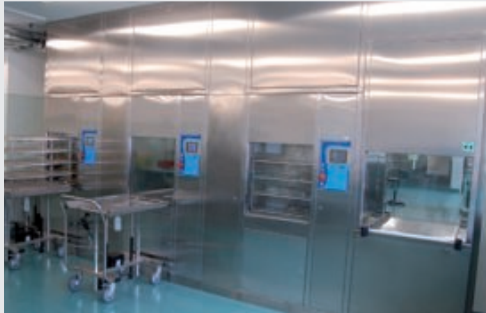
Washing machines loading view
