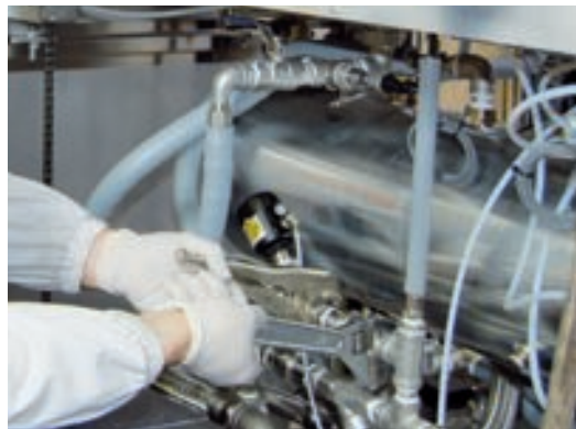
Stainless steel internal piping
