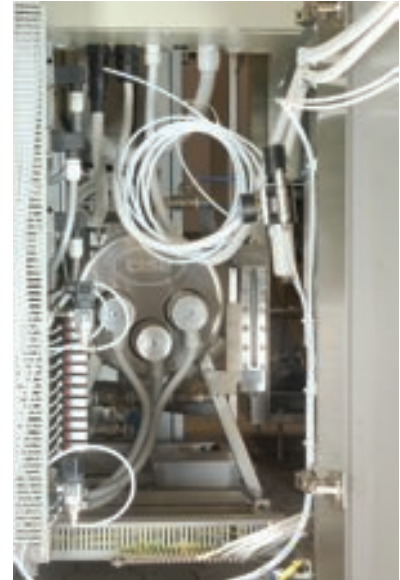
Steam generator energy saving
