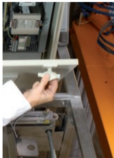
Electrical board with protection
