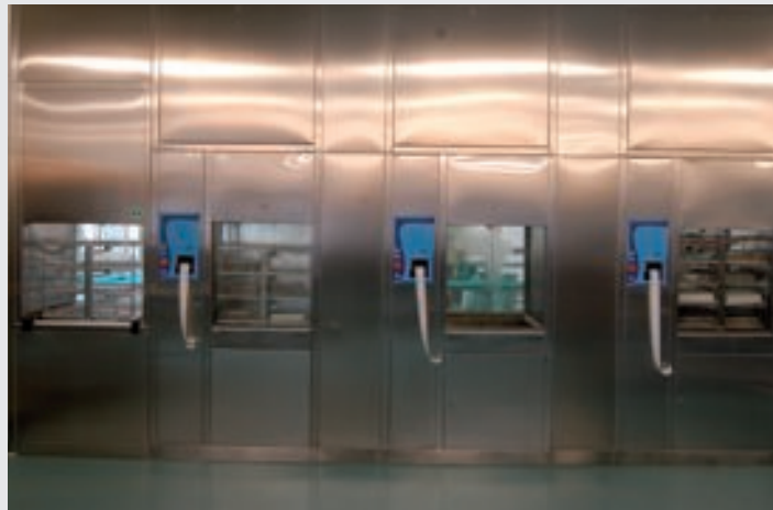
Washing machines unloading view
