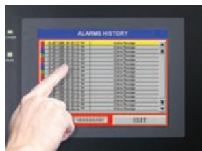
Touch Screen for alarms history
